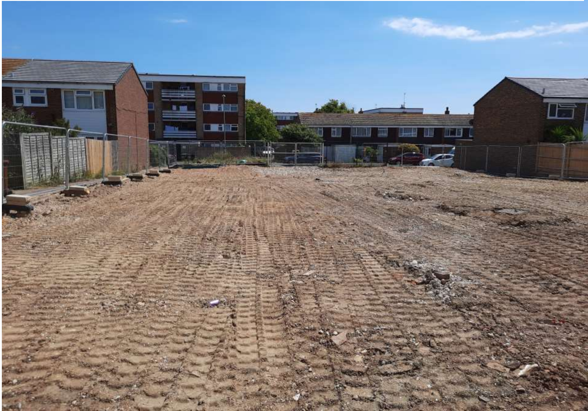
Site viewed from path to the rear (north) on Appledore Close
